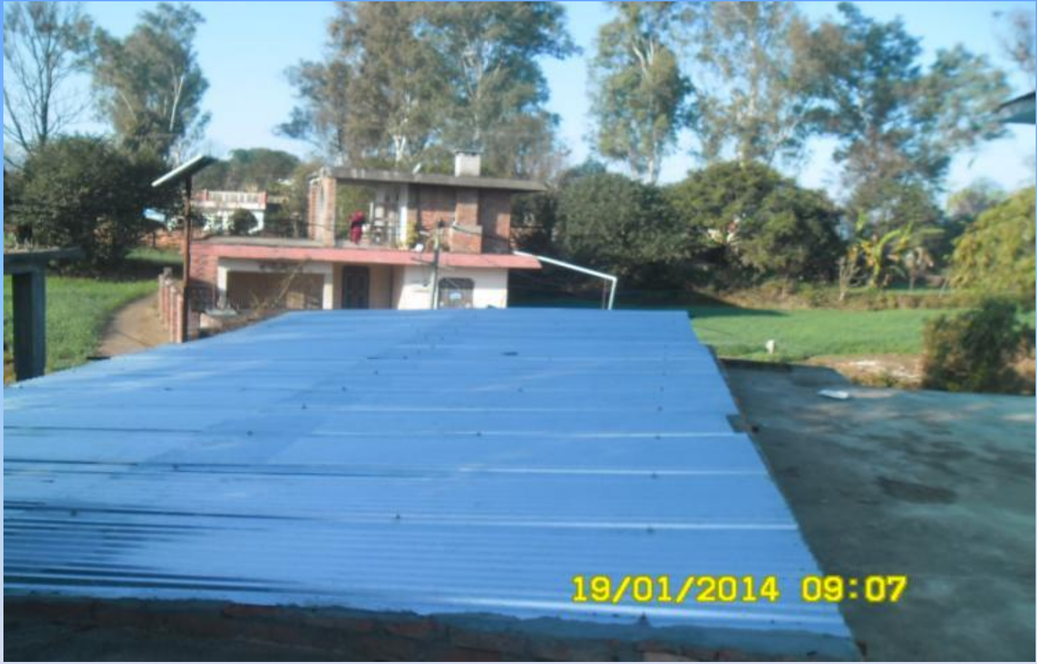
Top View of Panchayat Shed
